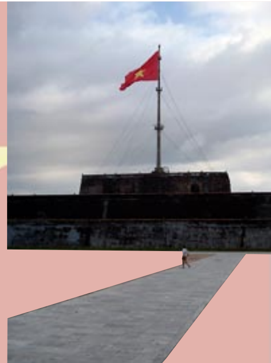
Above: Cot Co , or Flag Tower , first erected in 1809.
